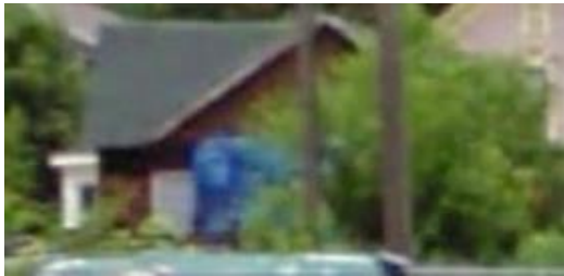
Google street view, June 2009. The blue tarp covers the area where the rear extension had been located.
