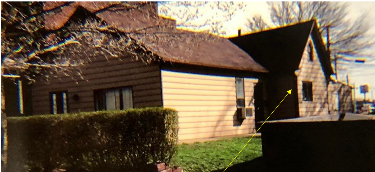
Designation photo – view from Wabash showing front and south-side elevations, 1984. HDAB.
