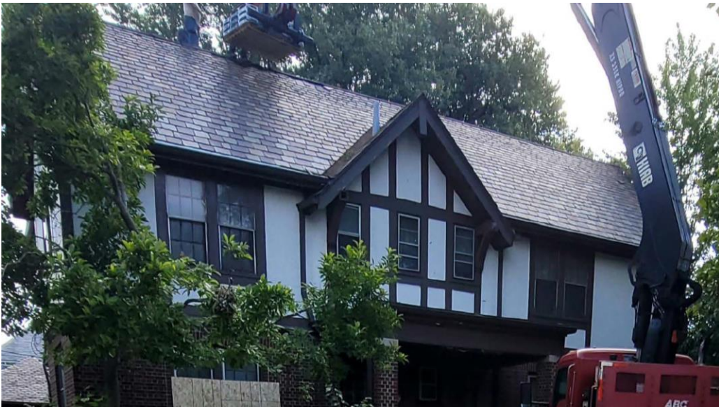
Photos of the roof submitted by applicant
