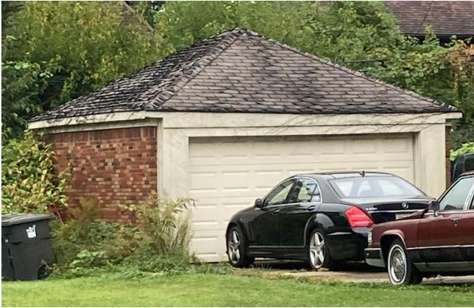
3777 Sturtevant garage, current condition. Staff photo taken on 9/28/2023
