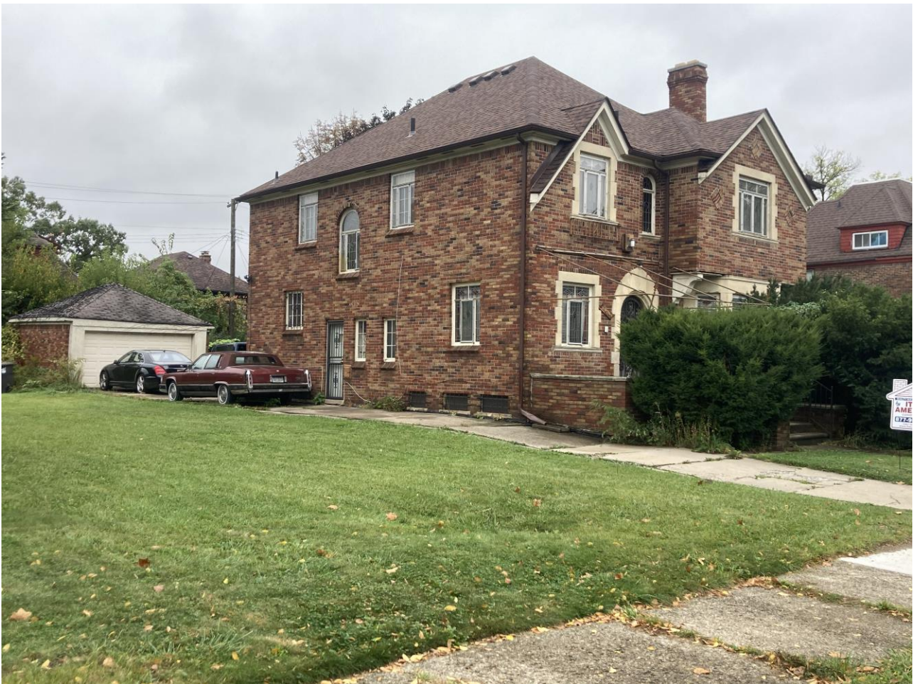
3769 Sturtevant (vacant lot to the left) and 3777 Sturtevant (house and garage), current condition. Staff photo taken on 9/28/2023
