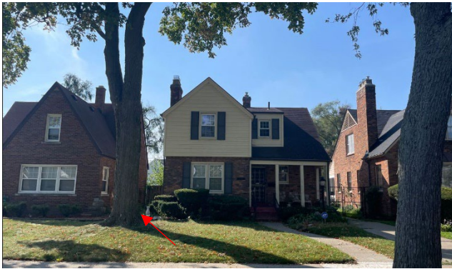
Site Photo 1, by Staff September 21, 2023: (East) front elevation, showing maple tree to the left of the house (arrow).
