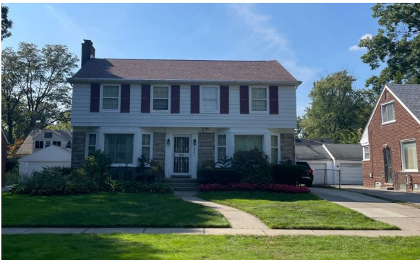
Site Photo 1, by Staff September 21, 2023: (East) front side
