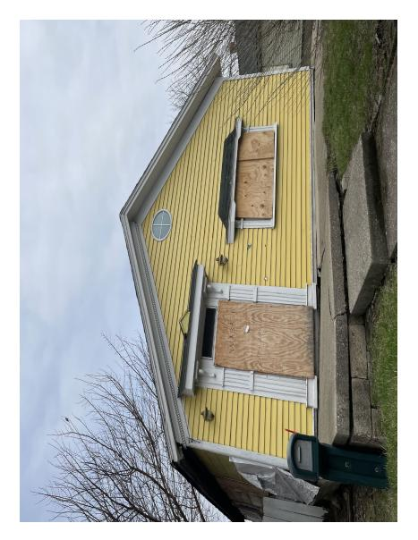
The cement porch, steps and grade will be removed to be flat with the public sidewalk, which is the way the neighbors both north and south are. The left side facing has the same siding but that only goes less than 1/4 of the way along the wall, that will be replaced as needed with identical wood siding to the front and right side facing (which is the south wall).. The framing
