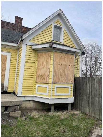
This addition was removed, and I believe was not original because the building materials were more modern, particle board and the framing was 18" on center and the 2x6 framing looked milled.
