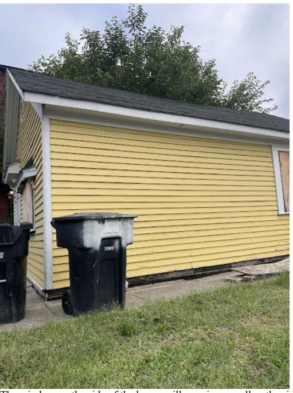
The window on the side of the house will remain, as well as the siding. The foundation will be removed and repaired/replaced with cement block.
