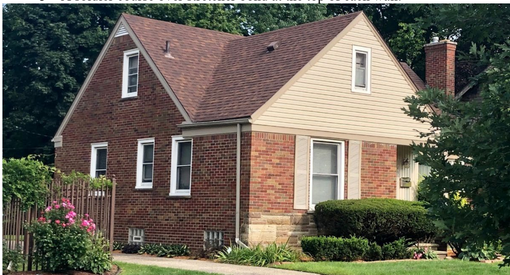
HDC staff photos, August 30, 2023. Above: North-side elevation. Right: South-side elevation.
