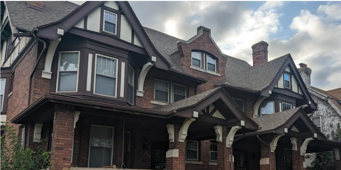
Example of open brackets on Arts and Crafts buildings. September 2023 photos by staff.
