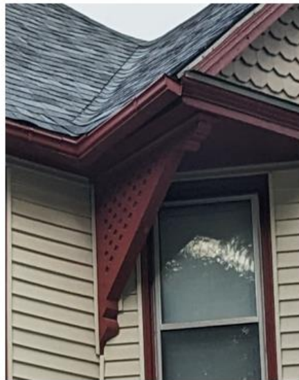
Open or perforated brackets on Queen Anne buildings. September 2023 photos by staff.
