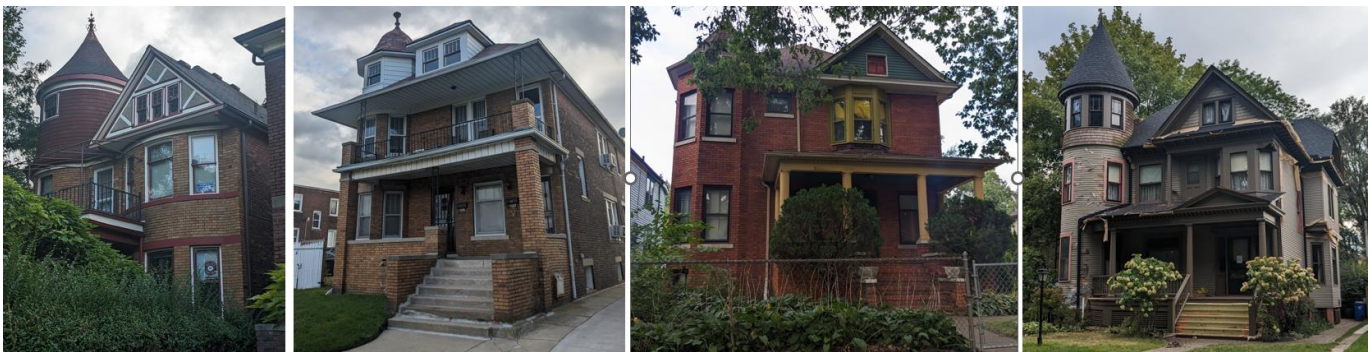
Above and next page: Buildings with towers in Hubbard Farms (only twelve are shown as the subject property is not depicted). September 2023 photos by staff.
