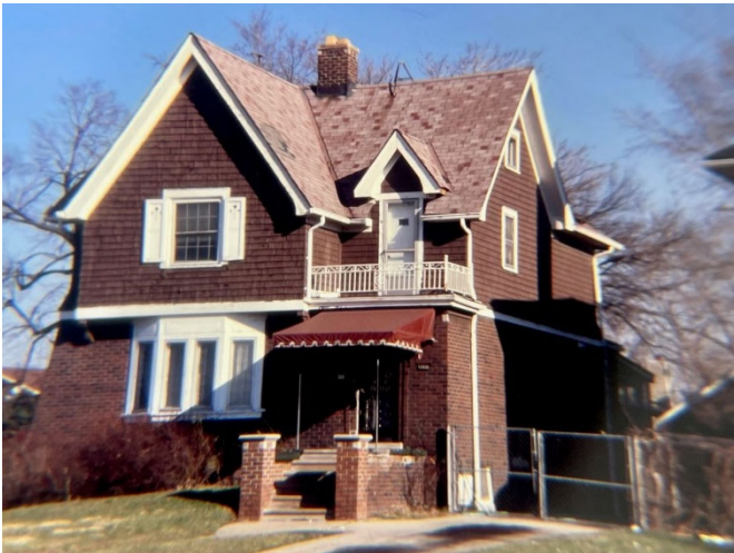
Designation Slide, 1999: (West) front/side elevation showing original condition.
