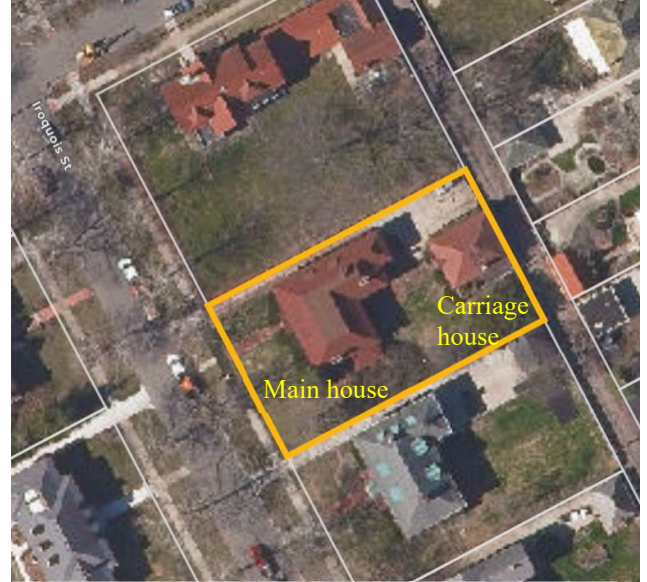
Aerial of Parcel # 14012174.
