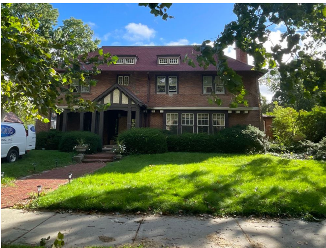
Site Photo 1, by Staff August 30, 2023: (West) front elevation of house, showing location of removed evergreen at southwest corner of the house, work completed without approval.
