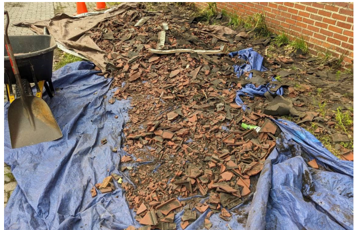
Site Photo 5, by Staff, August 1, 2023: Showing clay tile shattered on the ground in the alley.
