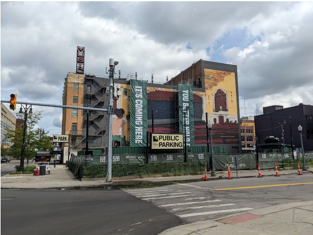
View of parcel from Randolph, looking east. Music Hall building in background. Staff photo, September 11, 2023.
