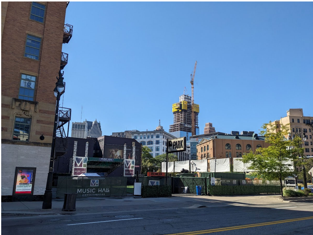
View of existing conditions at 300 Madison, looking towards the south. Staff photo, September 1, 2023.
