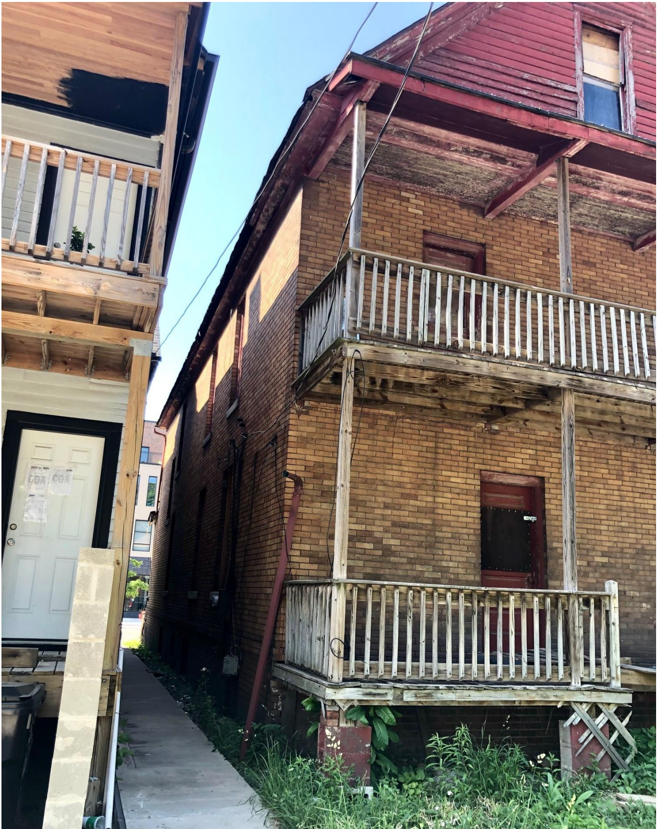
West elevation, looking north towards Kercheval from alley. Staff photo, May 30, 2023.
