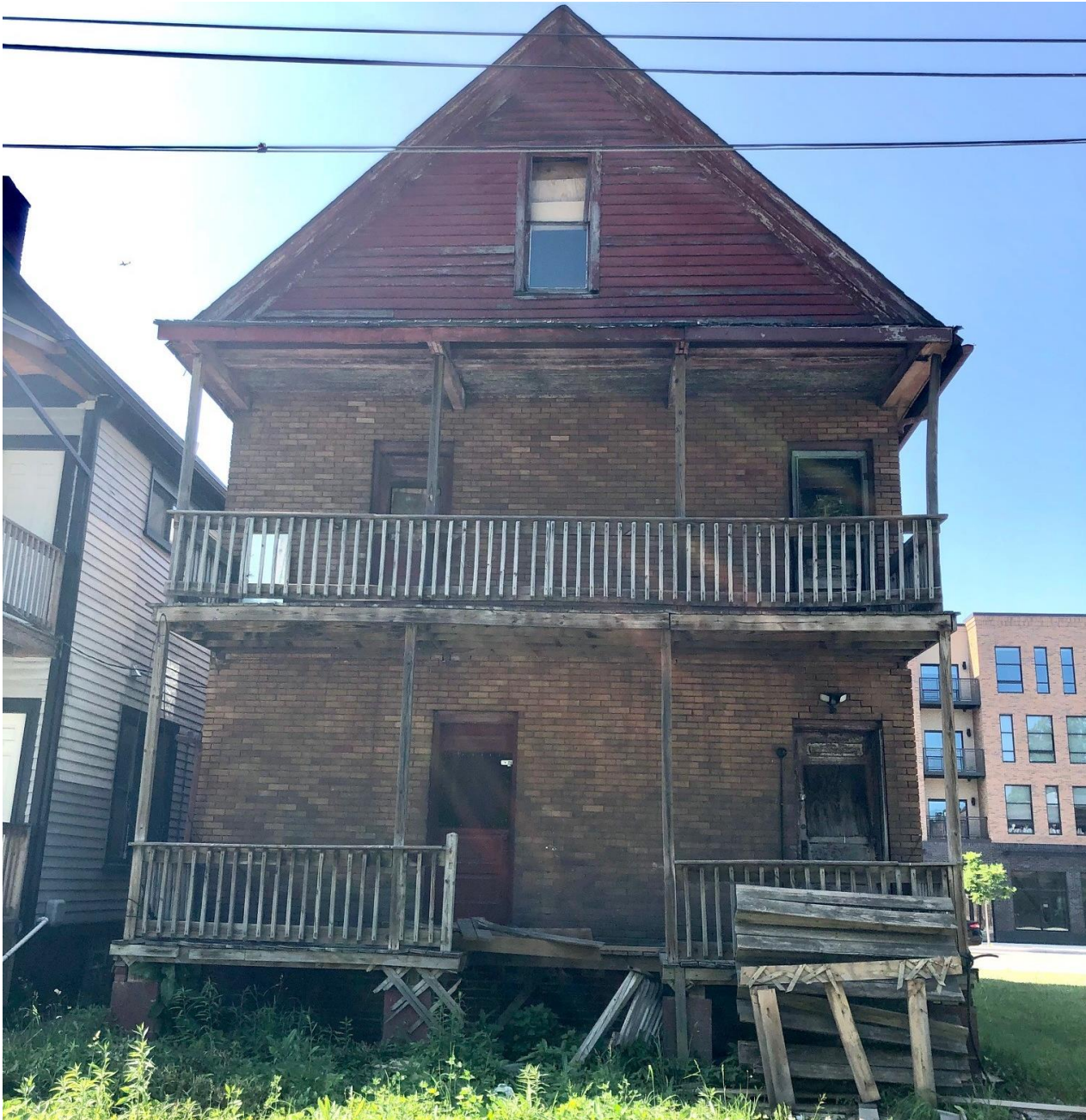
Rear elevation. Staff photo, May 30, 2023.
