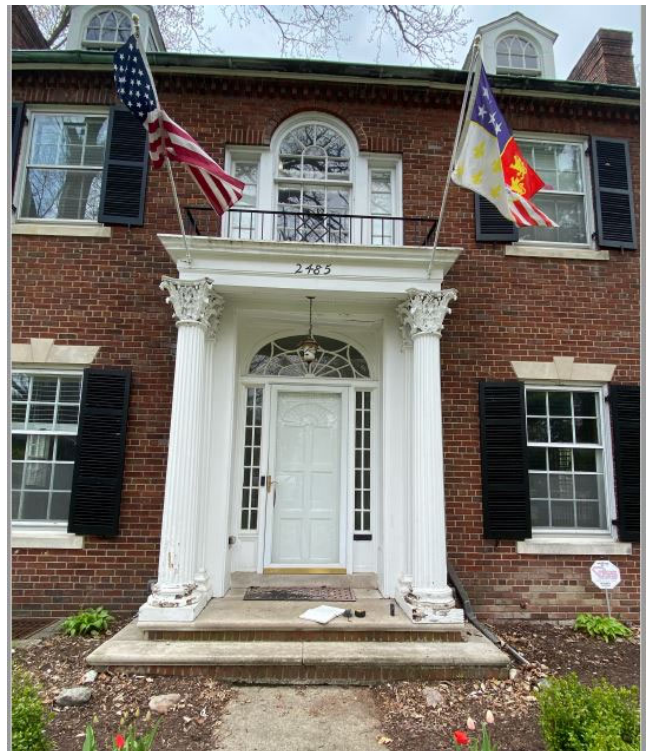
Site Photo 3, by Applicant: (East) front porch existing conditions.
