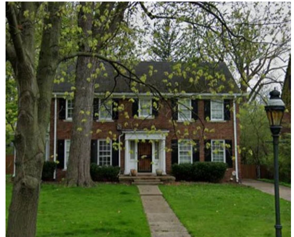
Site Photo 5, by Google Street May, 2019: 2211 Burns
