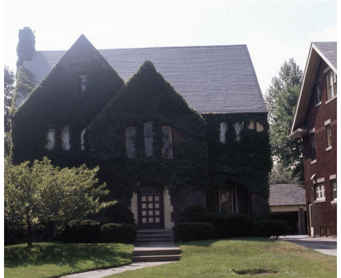
Site photo 4, 2135 Boston designation Image, 1974: (North) front elevation showing the 2325 Boston garage at rear.
