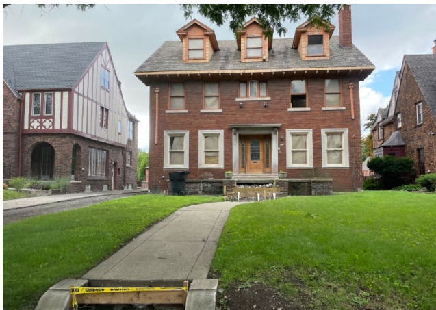
Site Photo 1, by Staff July 18, 2023: (North) front elevation.
