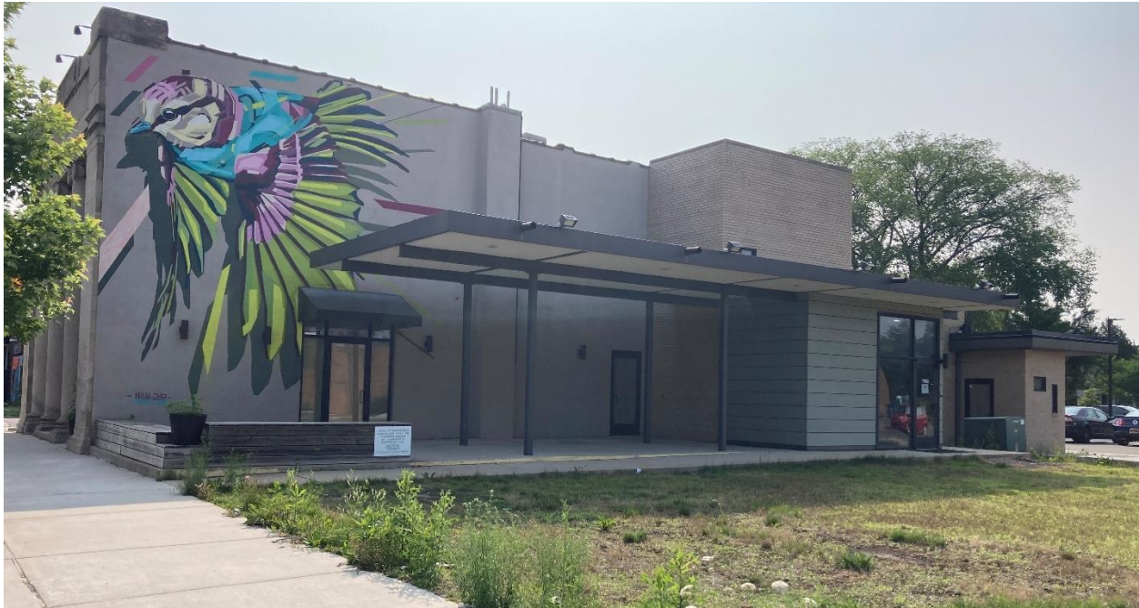
West elevation, current appearance, staff photo taken 7/3/2023. Note that the canopy, concrete pad, and small, one-story, fiber cement clad wing were installed during the 2015 building renovation. Note that stucco clads the majority of this elevation while buff brick cladding is located at the two-story ca. 1960s stair addition. Also, note the lack of historic ornamentation/decorative details at this elevation.
