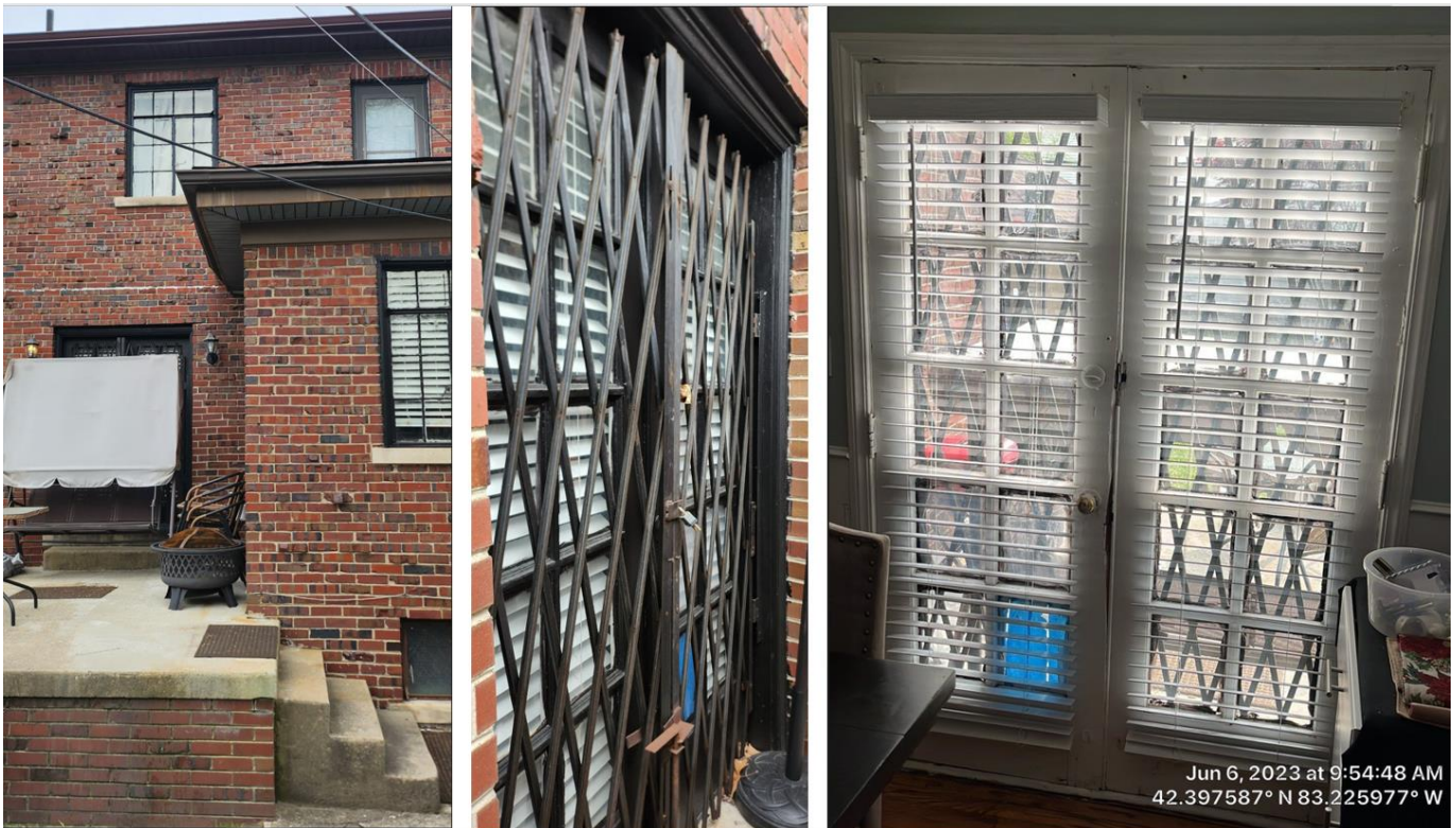
Existing door. Photos provided by applicant.
