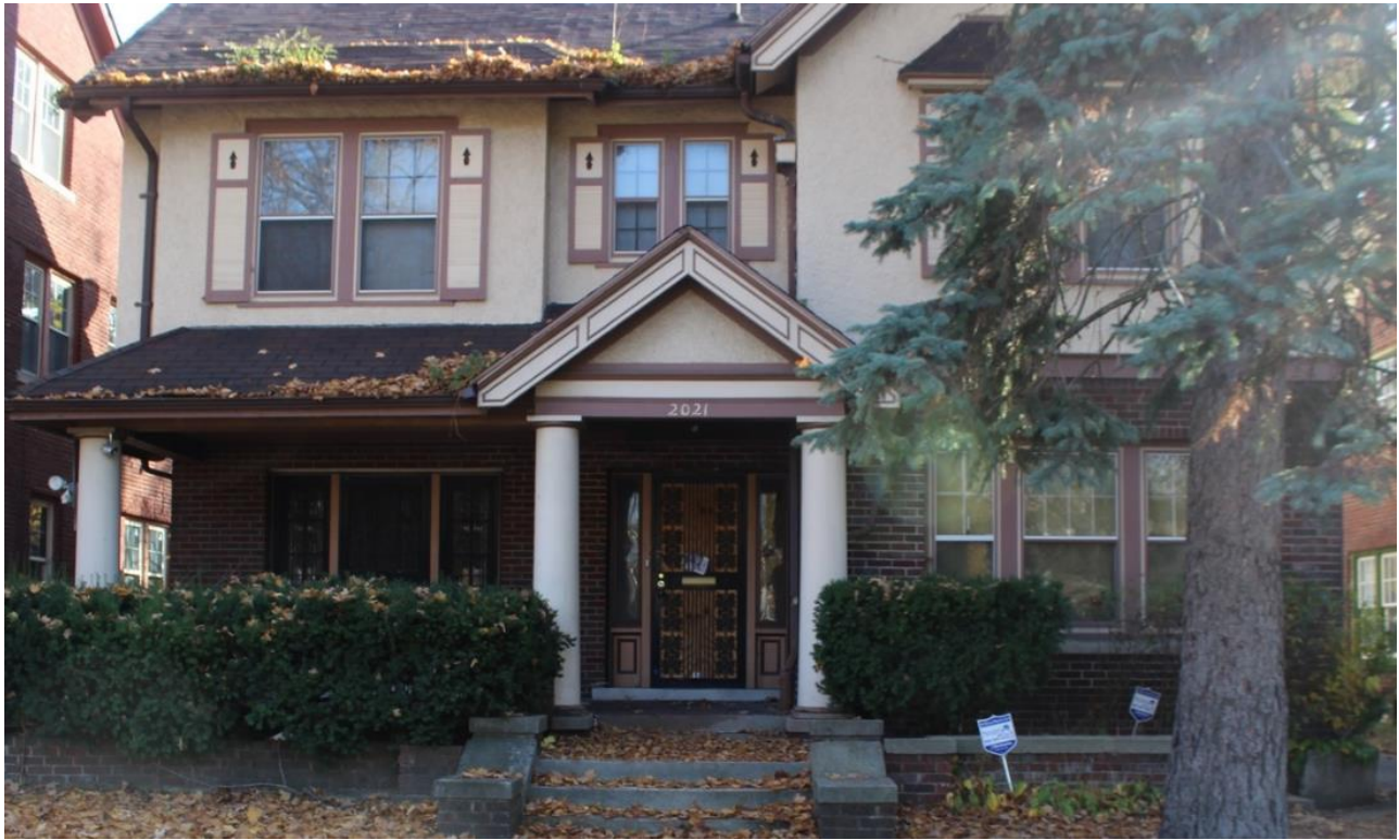
Appearance prior to the unapproved window replacement. Photo provided by applicant
