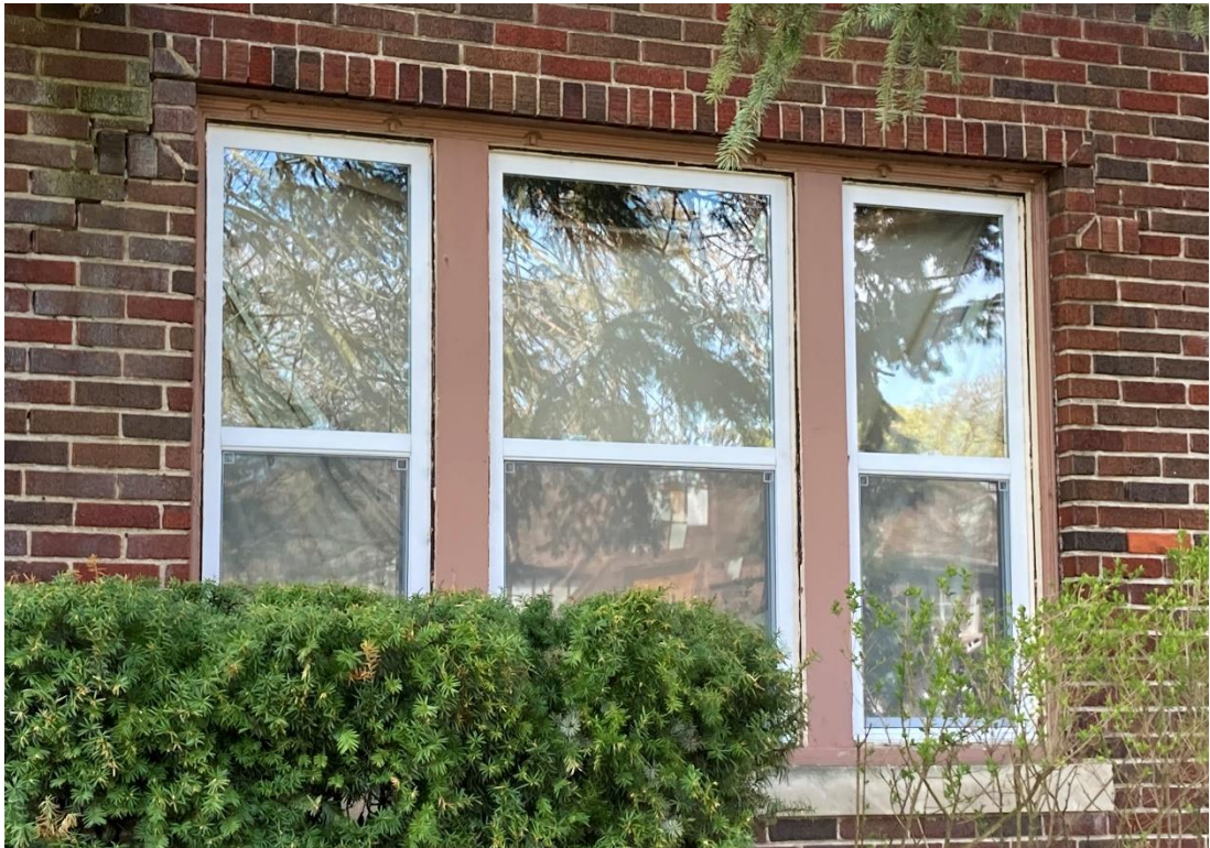
Existing conditions, photos taken by HDC staff on 4/23/2023. Note newly installed, 1/1 vinyl windows and remaining historic wood trim
