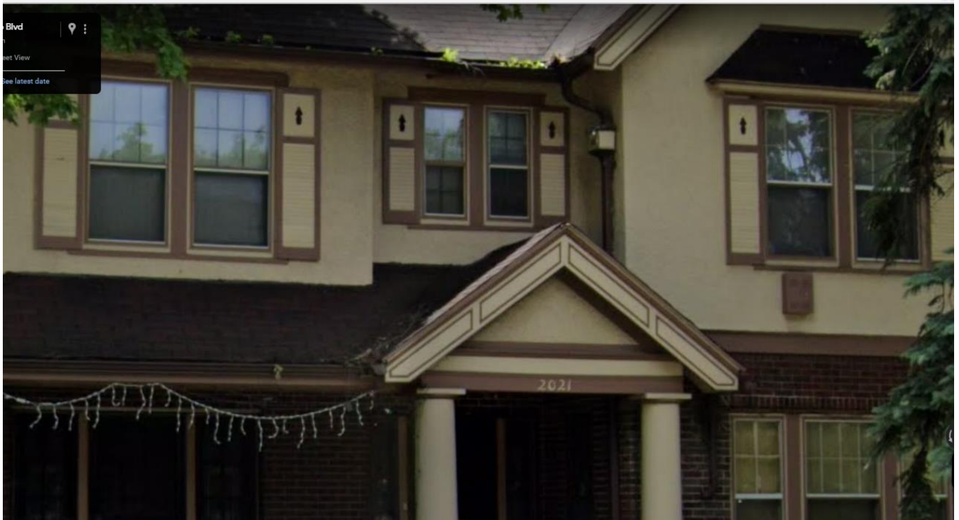
Appearance in 2019, prior to the unapproved window replacement (Google Streetview). Showing original wood windows
