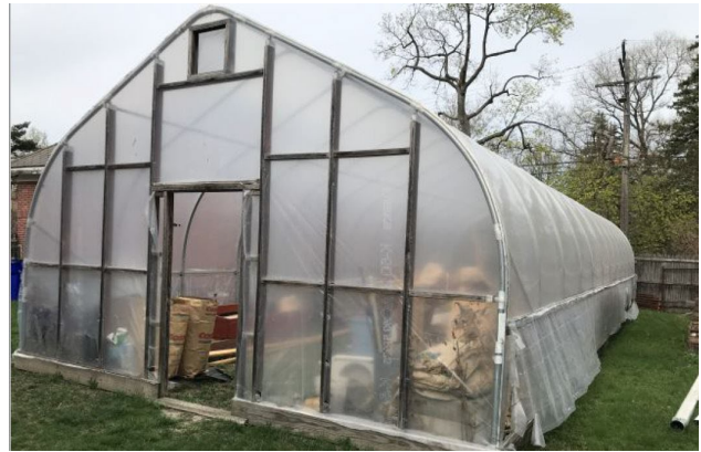
Site Photo 4, by Applicant, showing completed construction of hoophouse.
