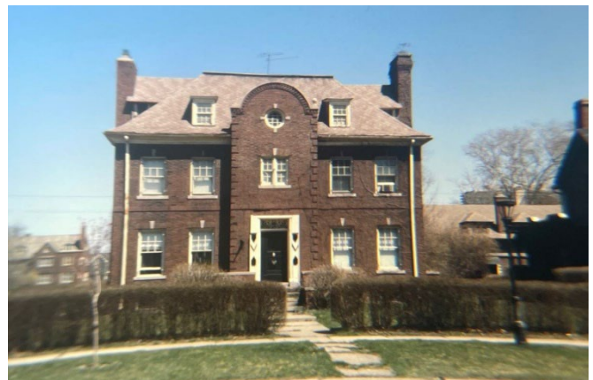
Site Photo 2, Designation Slide April 22, 1980: front elevation (west).
