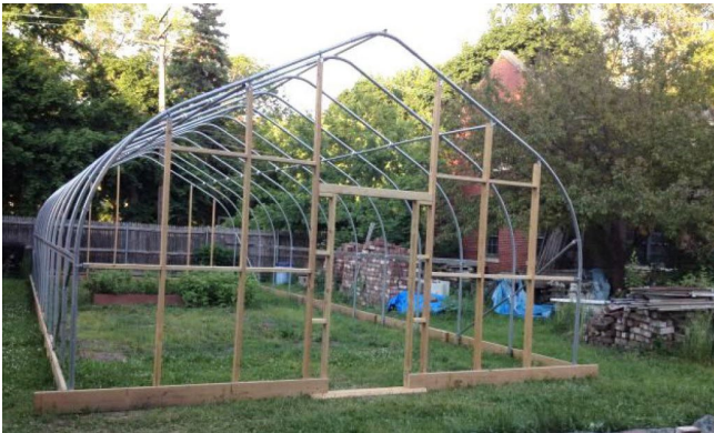
Site Photo 3, by Applicant, showing hoophouse framing.
