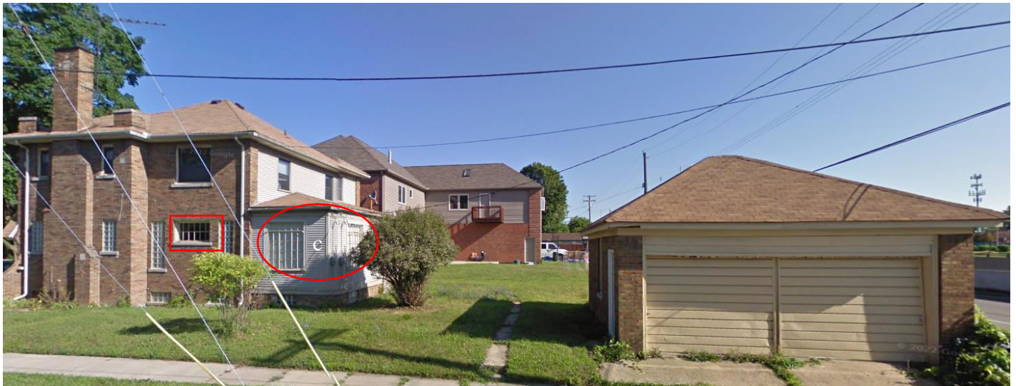
2009 Google Streetview image. Note the presence of steel casement windows at the casement windows at the rear wing's first story and the side elevation's first story. Also a rear deck and gate is not present in 2009 and the garage doors are different from the current single overhead door.
