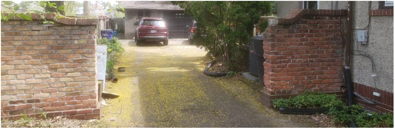
Existing wall opening. Image from application, cropped by staff.
