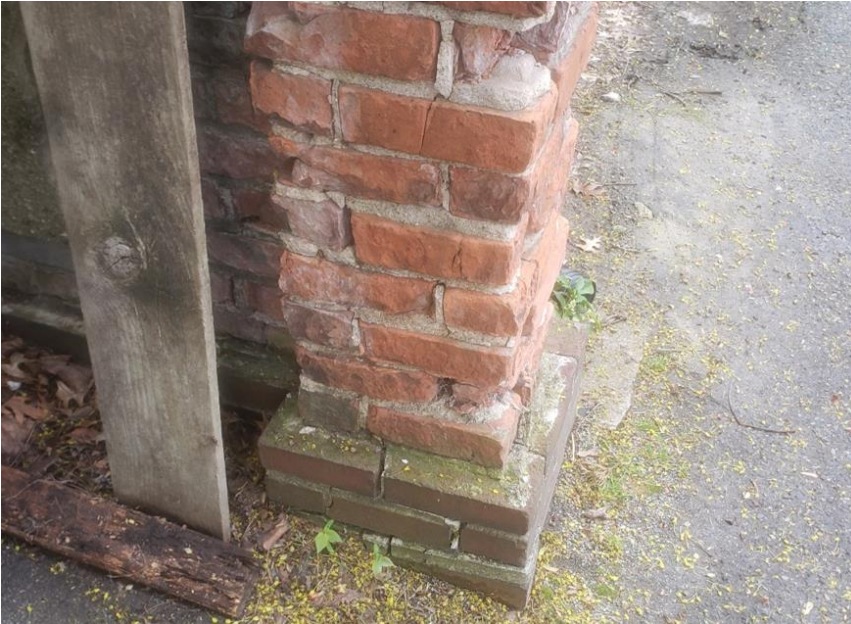
Interior view of southernmost pier. Image from applicant.
