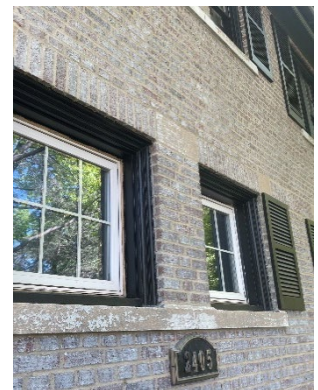
Site Photo 8, by Staff, May 24, 2023: (Northeast) side elevation, showing removed paint surface from brick and
