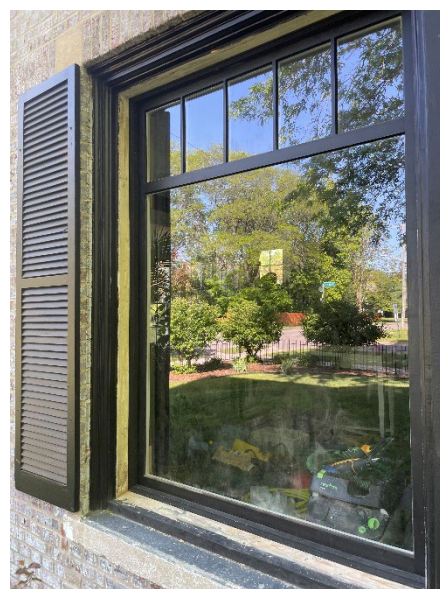
Site Photo 5, by Staff May 24, 2023: (Northeast) side elevation, detail of window #6 showing what appears to be a newly constructed wood window.
