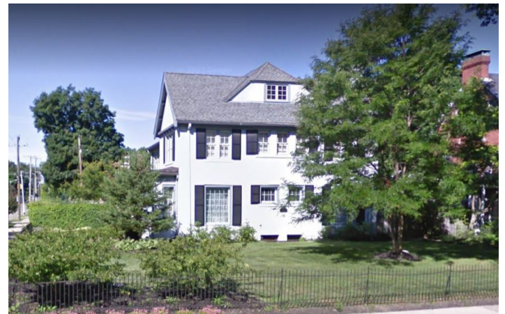
Site Photo 4, by Google Streetview, July 2009: (Northeast) side elevation, showing original and vinyl windows (by previous owner), and painted brick.
