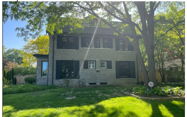
Site Photo 2, by Staff May 24, 2023: (Northeast) side elevation, showing three white vinyl windows that were previously installed by a former owner and replaced by current owner before June 5, 2023. The other windows were replaced by the current owner, replacing vinyl windows.
