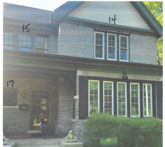
Figure 2, by Applicant: (Southeast) front elevation, showing existing vinyl windows #16.
