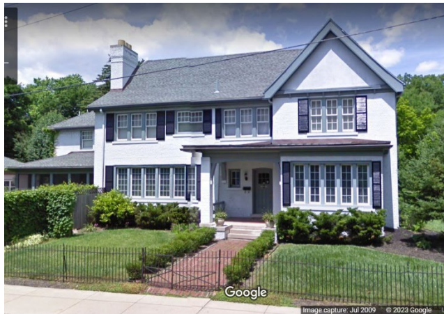
Site Photo 3, by Google Streetview, July 2009: (Southeast) front elevation, showing original and vinyl windows (by previous owner), painted brick, and original front door.
