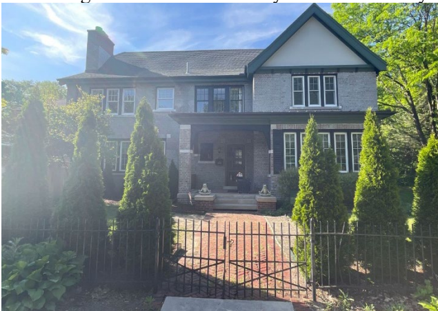
Site Photo 1, by Staff May 24, 2023: (Southeast) front elevation, showing vinyl windows from a previous owner and some wood windows.
