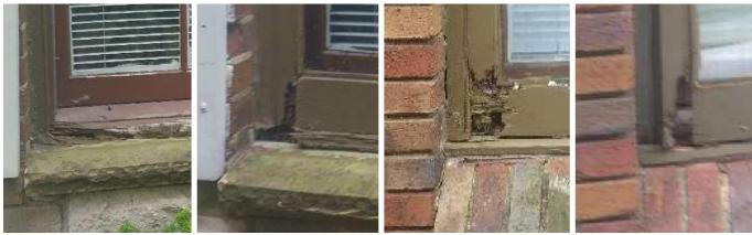
Deterioration of window frames and storm windows (no storm window is present on the leftmost image). Photos from application materials.
