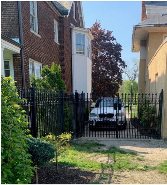
Gate meets southwest/rear corner of house.
