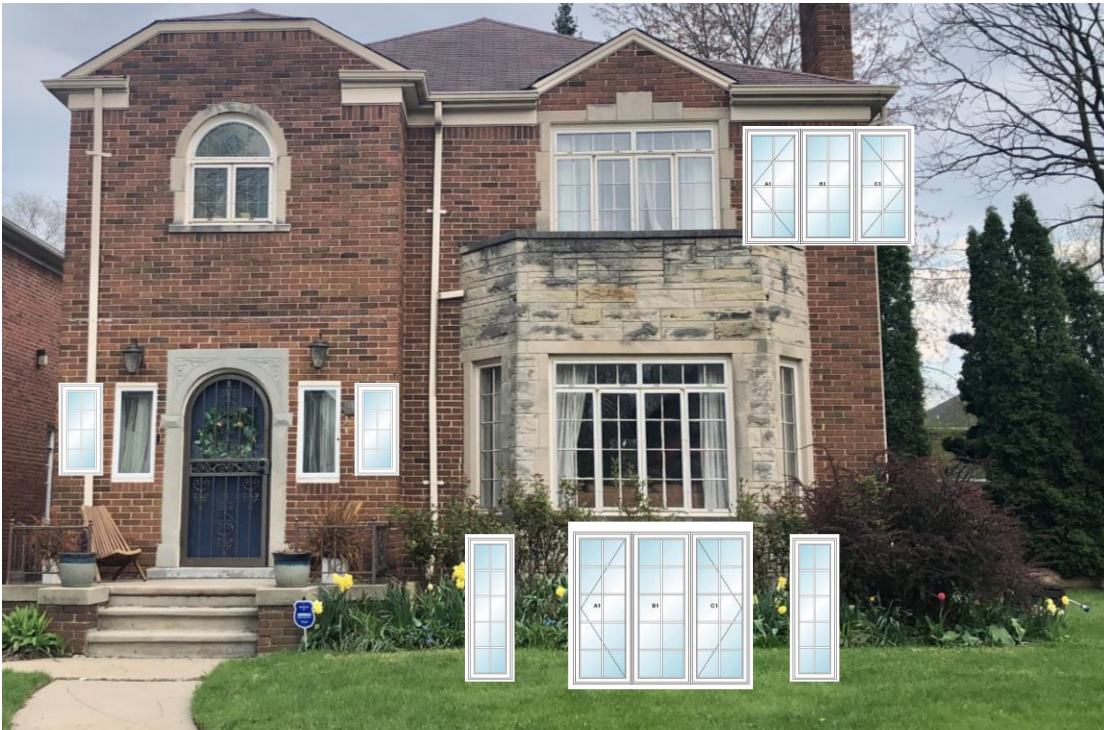
Staff photo, April 26, 2023. The rough opening width of the first and second floor openings are the same; the upper windows are approximately 12” shorter in height. The single casement side windows in the first floor bay would mimic the operation and design of the existing windows, whereas the other openings change operation and appearance.
