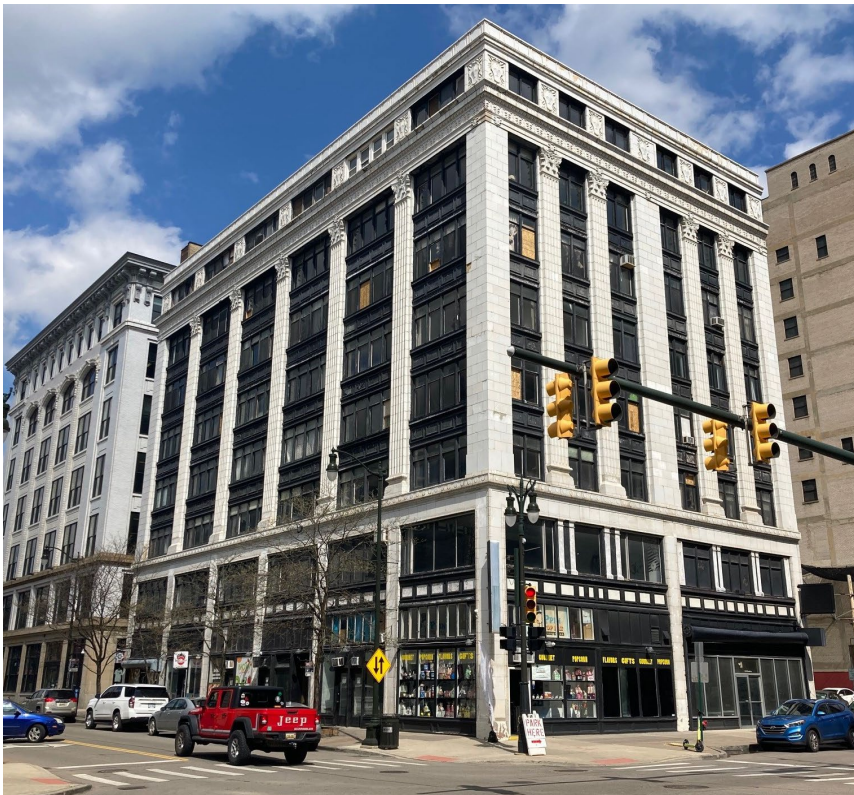
Figure 1: 206 E. Grand River Ave., looking east.
