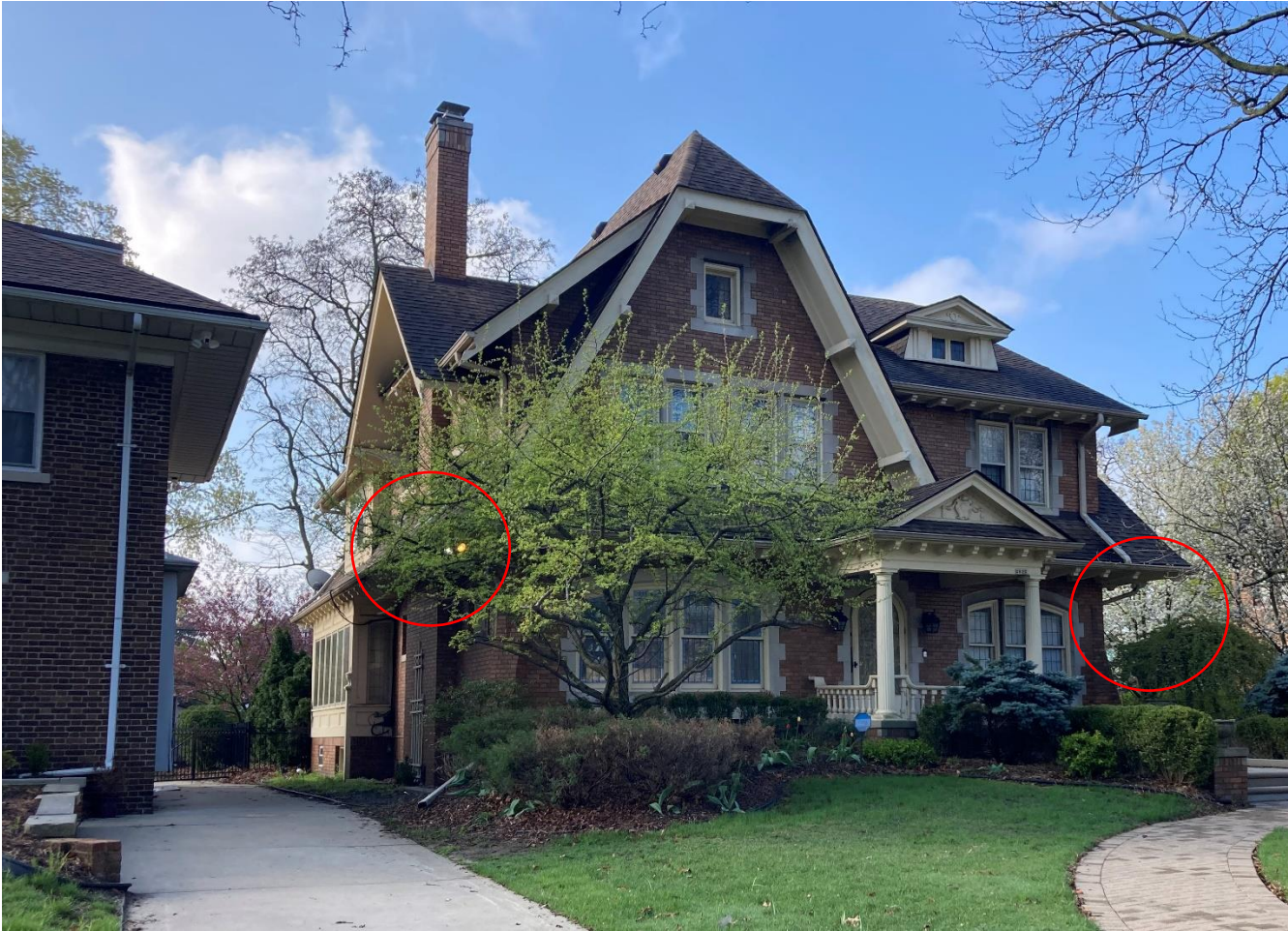
At 2035 W. Boston, two extant security lights at the at front within the eaves, 4/23/2023 staff photos
