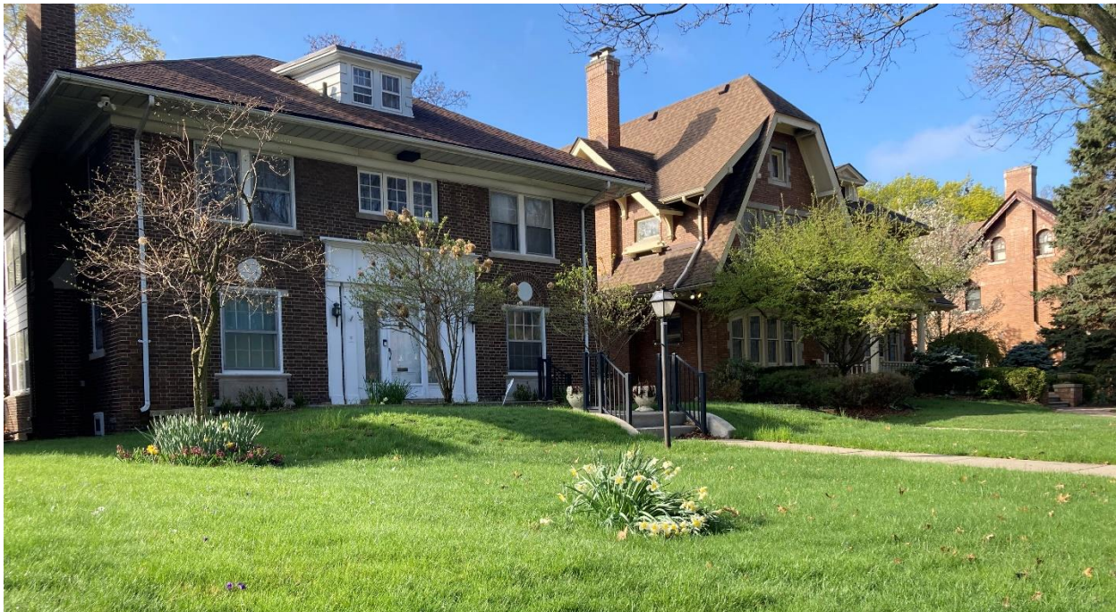
2027 W. Boston (left) and 2035 W. Boston (right) current appearance facing southwest, photo taken by staff on 4/23/2023
