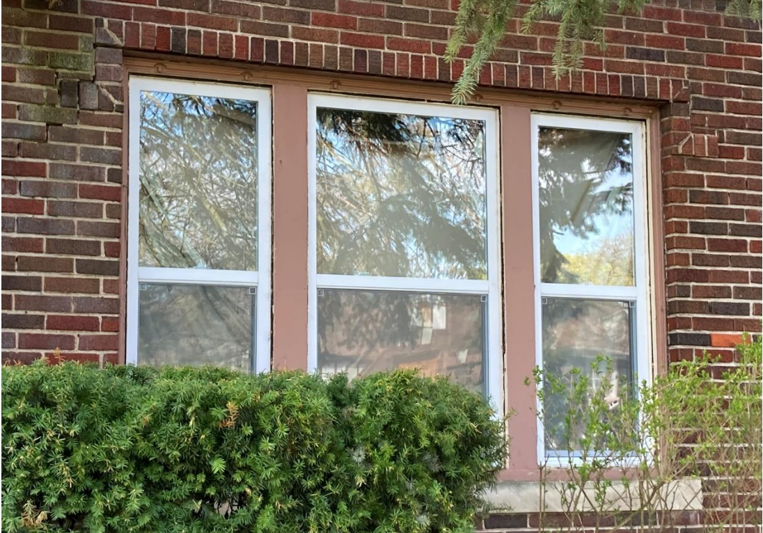
Existing conditions, photos taken by HDC staff on 4/23/2023. Note newly installed, 1/1 vinyl windows and remaining historic wood trim
