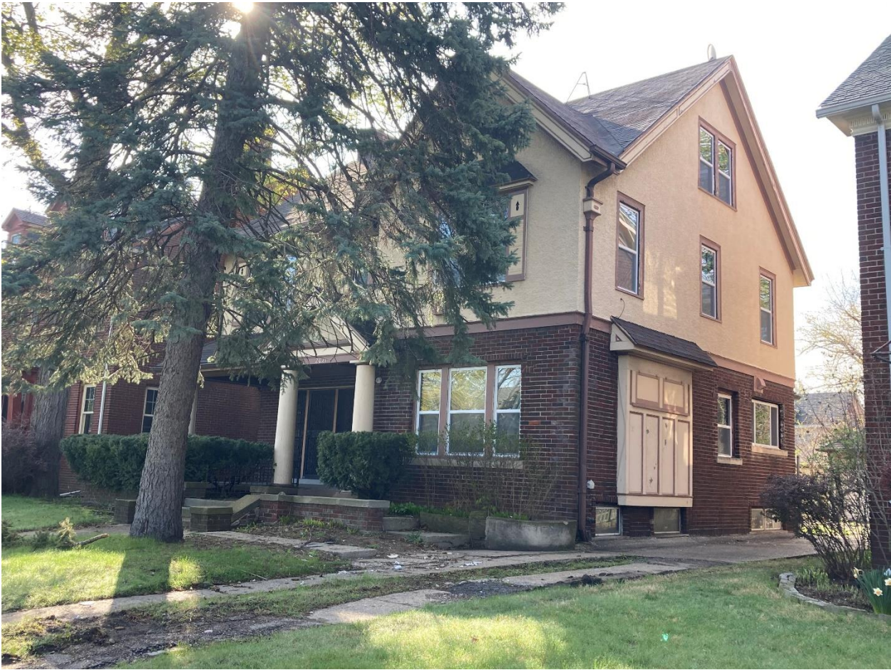
Existing conditions, photos taken by HDC staff on 4/23/2023. Note newly installed, 1/1 vinyl windows
