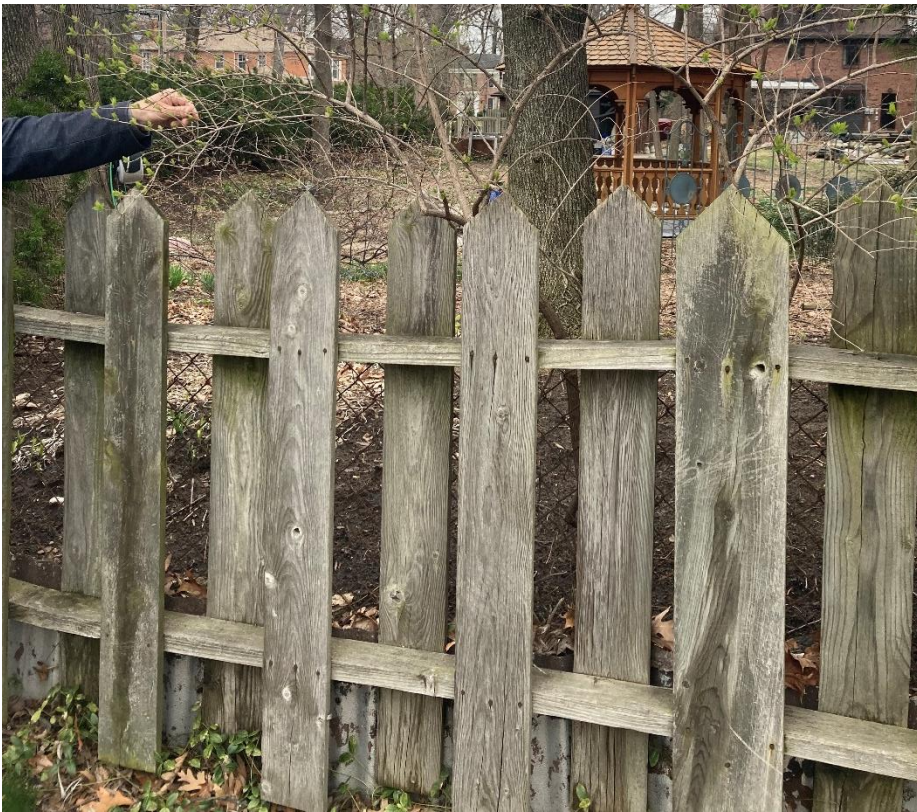
Existing fencing proposed for replacement (staff photo taken 4/4/2023)
