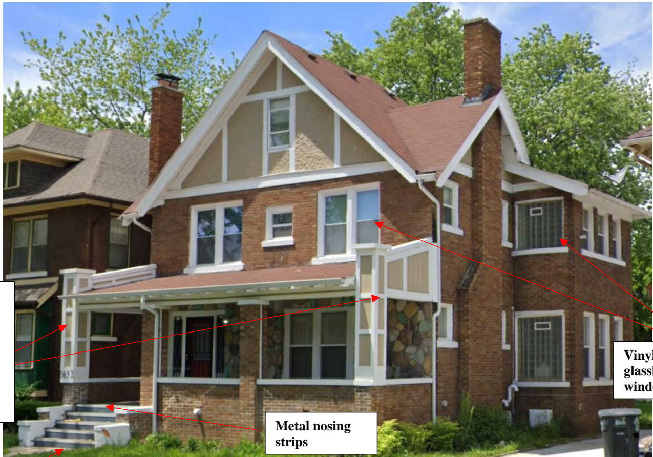
Google Streetview image of 1652 Edison, appearance in 2017 after the unapproved work
