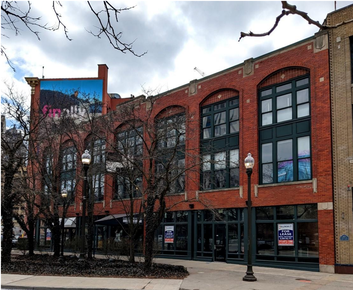
View from intersection of Randolph St. looking west towards front façade of building. Note alternating fixed and operable storefronts. February 2023 photo by staff.
