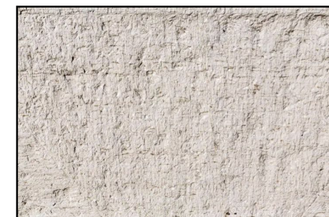
LIMESTONE SLAB - TRIM, BASE AND CORNICE
