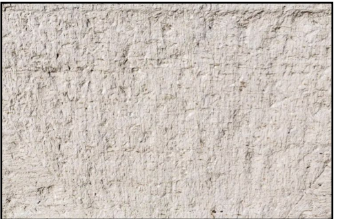
LIMESTONE SLAB - TRIM, BASE AND CORNICE
