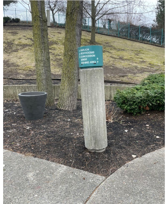
Site Photo 5, by Staff March 2, 2023: (North) entrance showing pylon #5.
