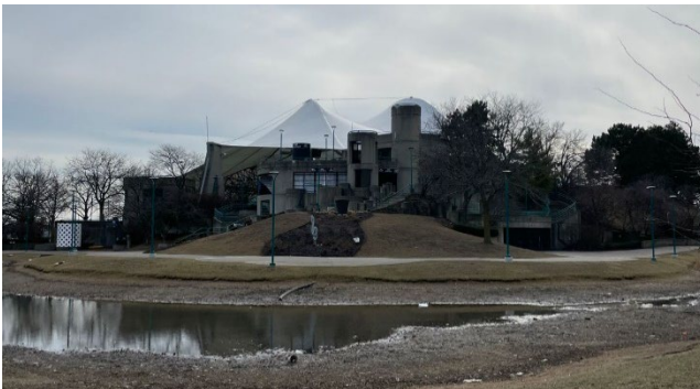
Site Photo 1, by Staff February 20, 2023: (North) Front elevation, showing evergreens to be saved from demolition to the right.
