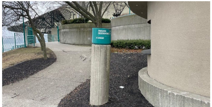
Site Photo 2, by Staff March 2, 2023: (East) Pavilion entrance showing pylon #11 and distinctive character-defining concrete surface finish treatment that complements the architectural composition of the site.
