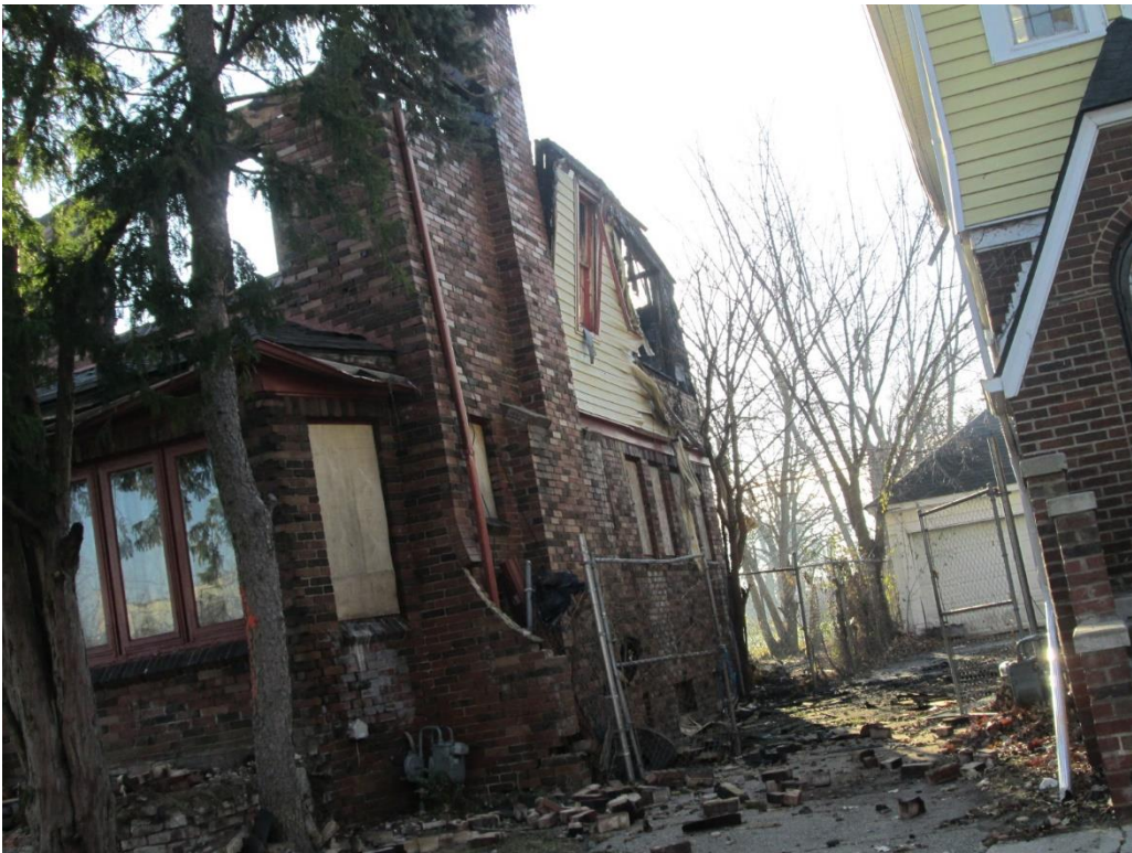
BSEED photos, taken in November 2022, prior to emergency demolition
