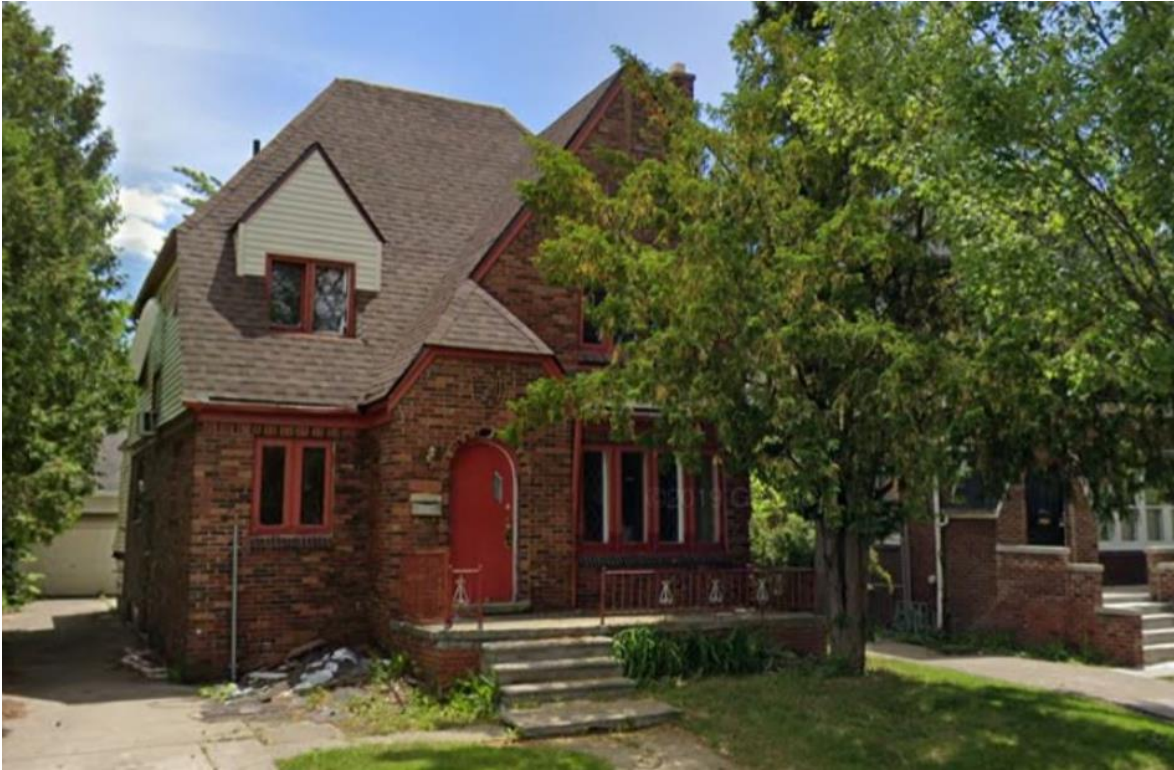
Google Streetview image, 2019 showing conditions prior to fire damage
