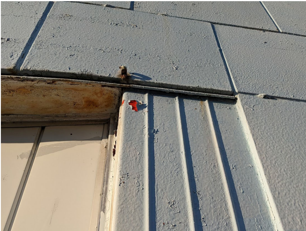
Detail view of porcelain enamel panels to immediate right of storefront opening; note original red finish visible. Staff photo, January 24, 2023.
