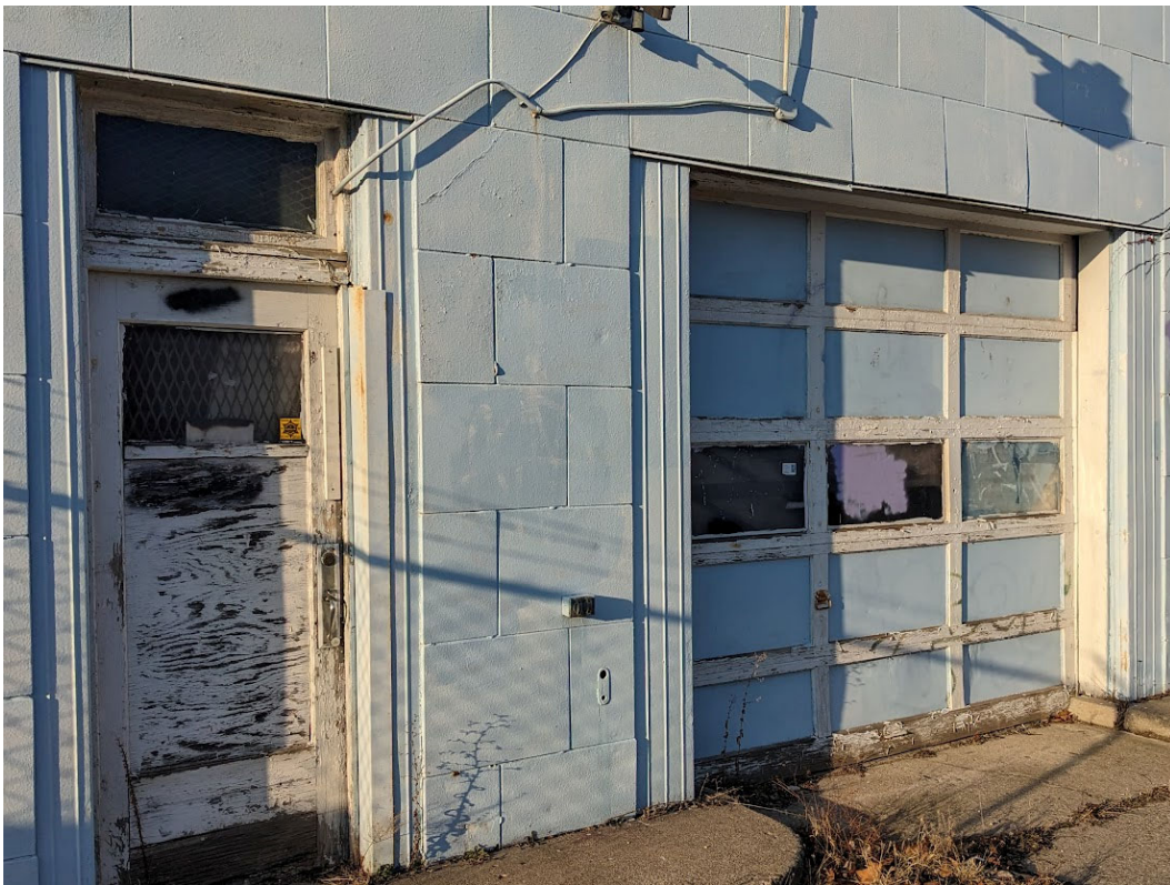
View of porcelain enamel panel system and original doors at south elevation; note the vertically oriented “drapes” positioned at either side of the openings, which are part of the panel system. Staff photo, January 24, 2023.
