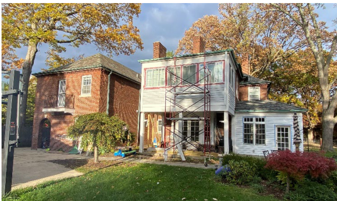
Site Photo 3, by Applicant: (Southeast) rear elevation showing new windows and siding of upper "sleeping porch" and former screened porch.
