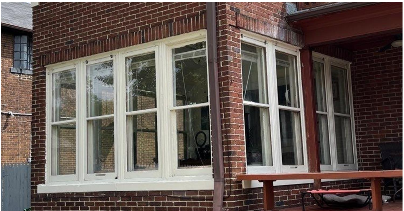
Image from application, cropped by staff. Additional interior and exterior photos are included in the submitted application materials.
