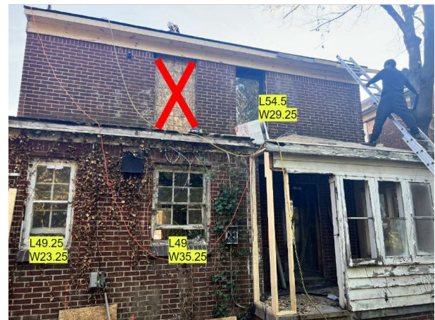
Site Photo 6, by Applicant 2022: (North) rear elevation showing proposed locations for new windows.
