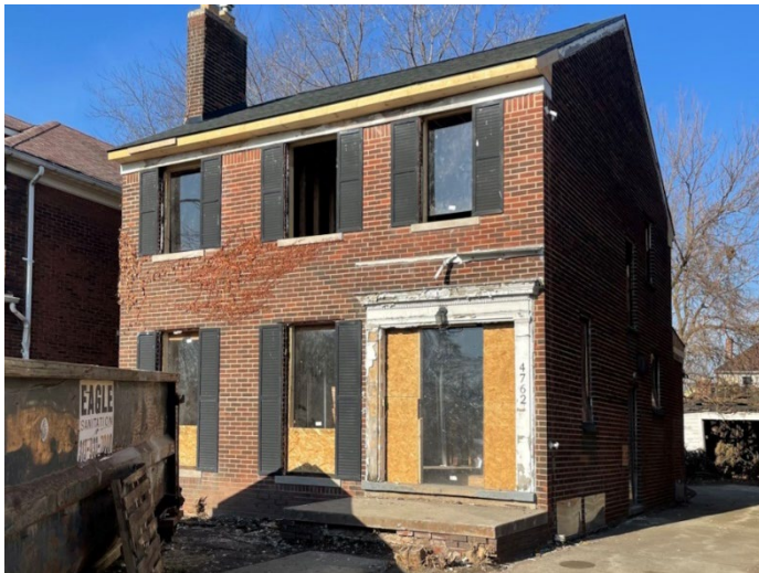
Site Photo 1, by Staff November.23, 2022: (South) front elevation.
