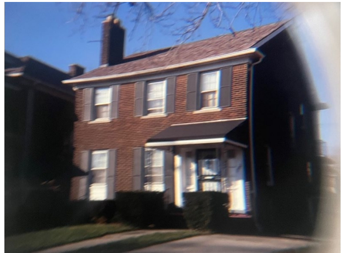
Designation Slide, 1999: (South) front/side elevation showing original windows, porch, entrance, and roof. Note greater eave depth.
