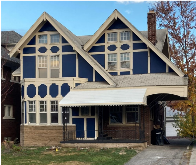
Figure 1: Current image of 2066 Atkinson Ave.
