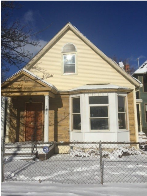
Figure 8: Dwelling before construction.
