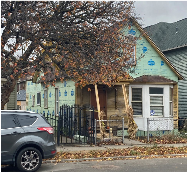
Figure 1: Current image of 1688 Bagley Ave.
