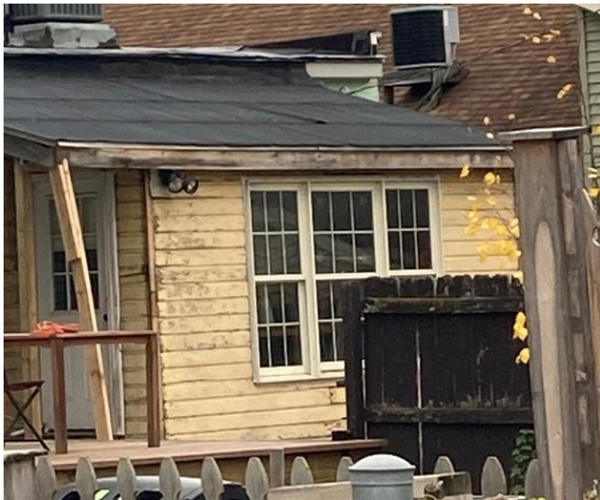
Figure 14: Ca. 1885 rear portion of the dwelling showing existing wood siding.
