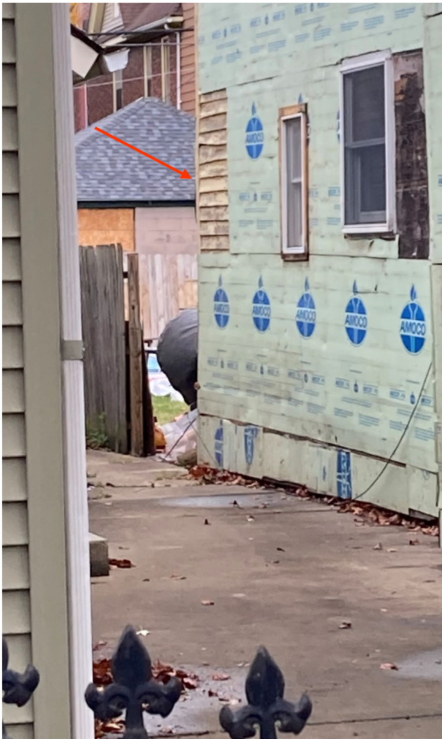
Figure 12: Wood siding on the western elevation
