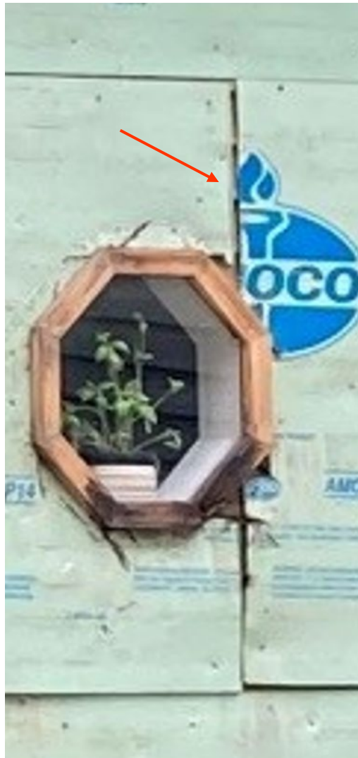
Figure 13: Wood siding under insulation, east elevation.
