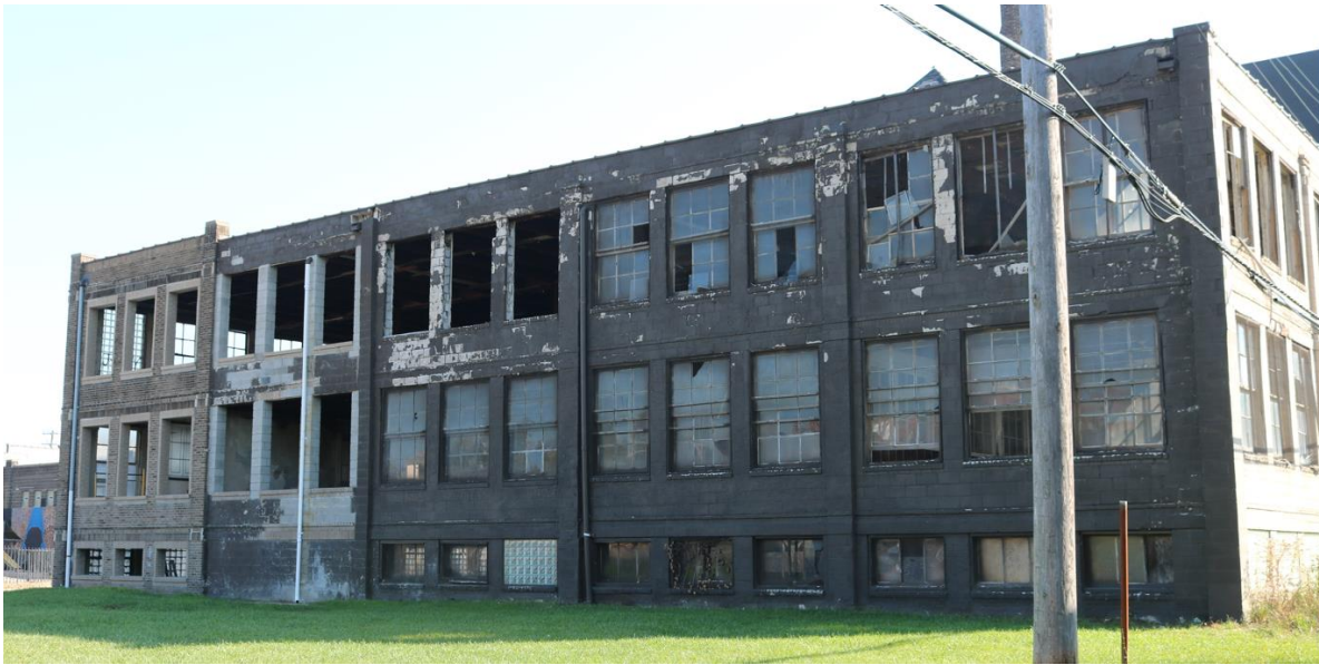
November 2022 photo by staff showing missing windows and one glass block window on the north elevation, work done without approval. Masonry repairs visible in the second bay from the left have likewise not received a Certificate of Appropriateness.
