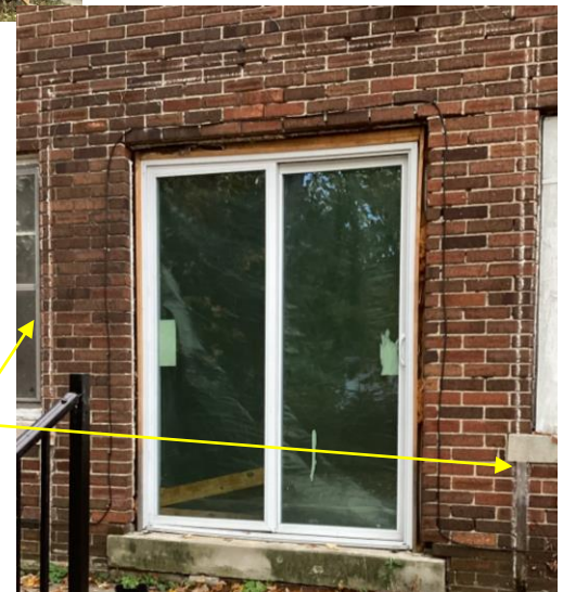
Applicant photos. Left: Stairs and wing walls. The recently poured concrete for the new railing is circled. Right: Ghost lines at rear door leading to open porch.
