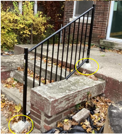
Applicant photos. Left: Stairs and wing walls. The recently poured concrete for the new railing is circled. Right: Ghost lines at rear door leading to open porch.
