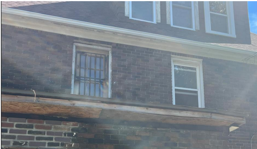
Photo from application shows historic fascias and soffits on the core block of the house, and fascias and soffits replaced by OSB and dimensional lumber on a rear ell.
