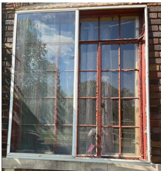
Historic steel window (typical of both windows on the front façade). Photo from application.
