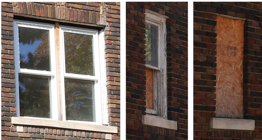
Examples of existing window openings. Left to right: Vinyl windows (note unpainted wood mullion), historic wood window, boarded-up opening. October 2022 photos by staff.
