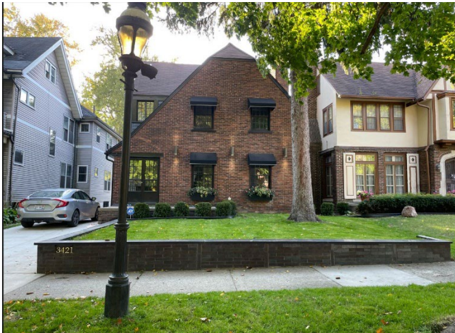
Site Photo 1, by Staff October 21, 2022: (Northeast) front elevation.
