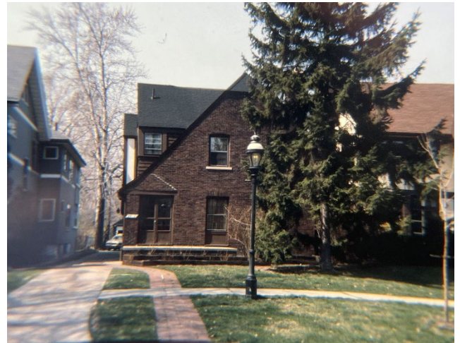
Site Photo2, designation photo 1980: (Northeast) front elevation.
