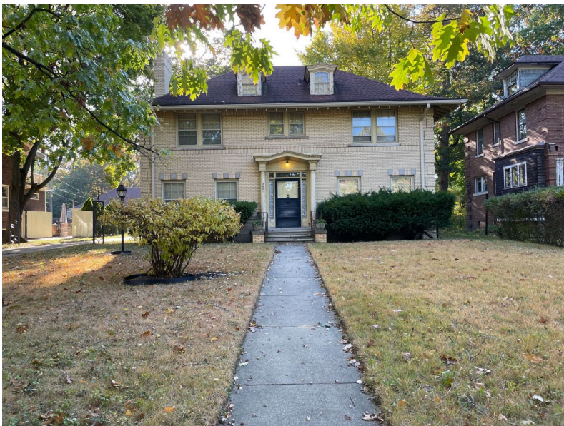
Site Photo 1, by Staff October 21, 2022: (Northeast) front elevation side
