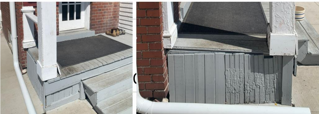
Rear porch. Photos by applicant.
