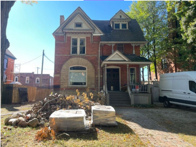
Site Photo 1, by Staff Sept.23, 2022: (North) front elevation.
