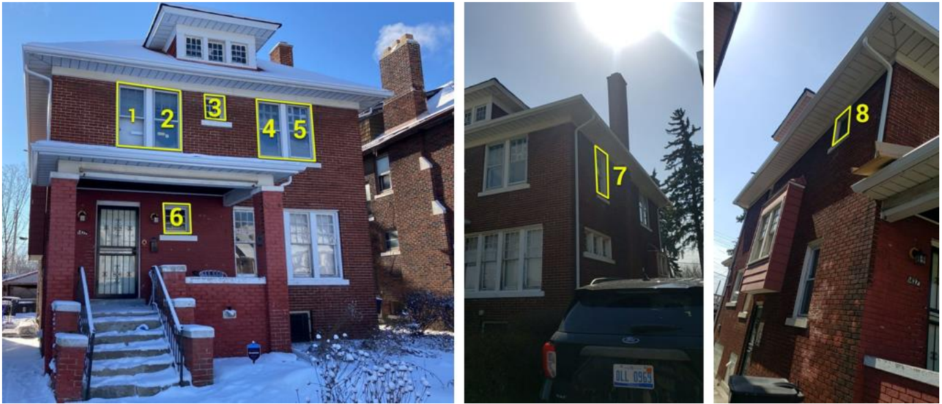
Eight windows proposed for replacement.
