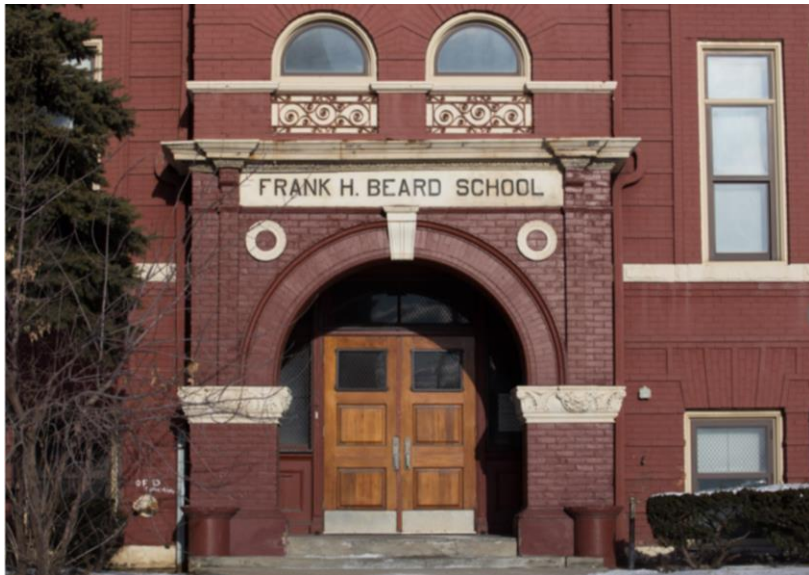
312 Waterman, conditions prior to fire, 2021
