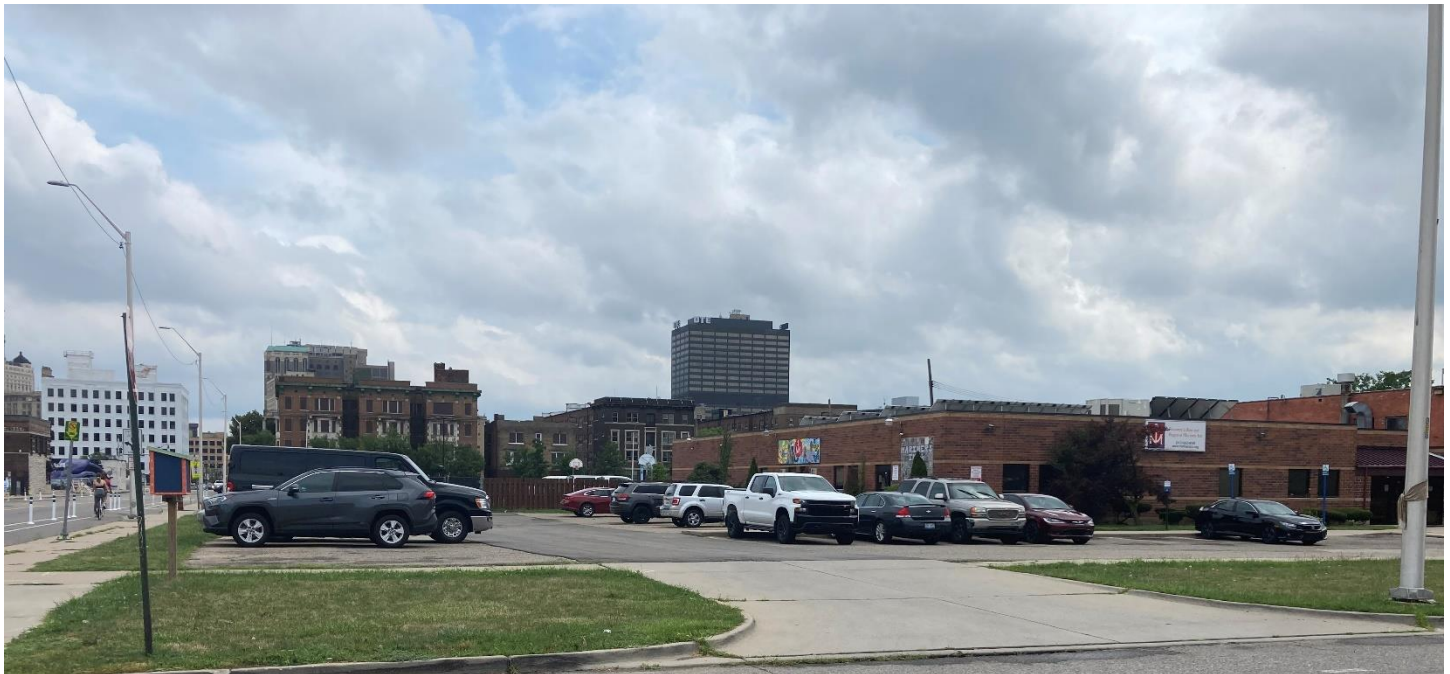
445 Ledyard, current appearance. Staff photo, taken 7/29/2022
