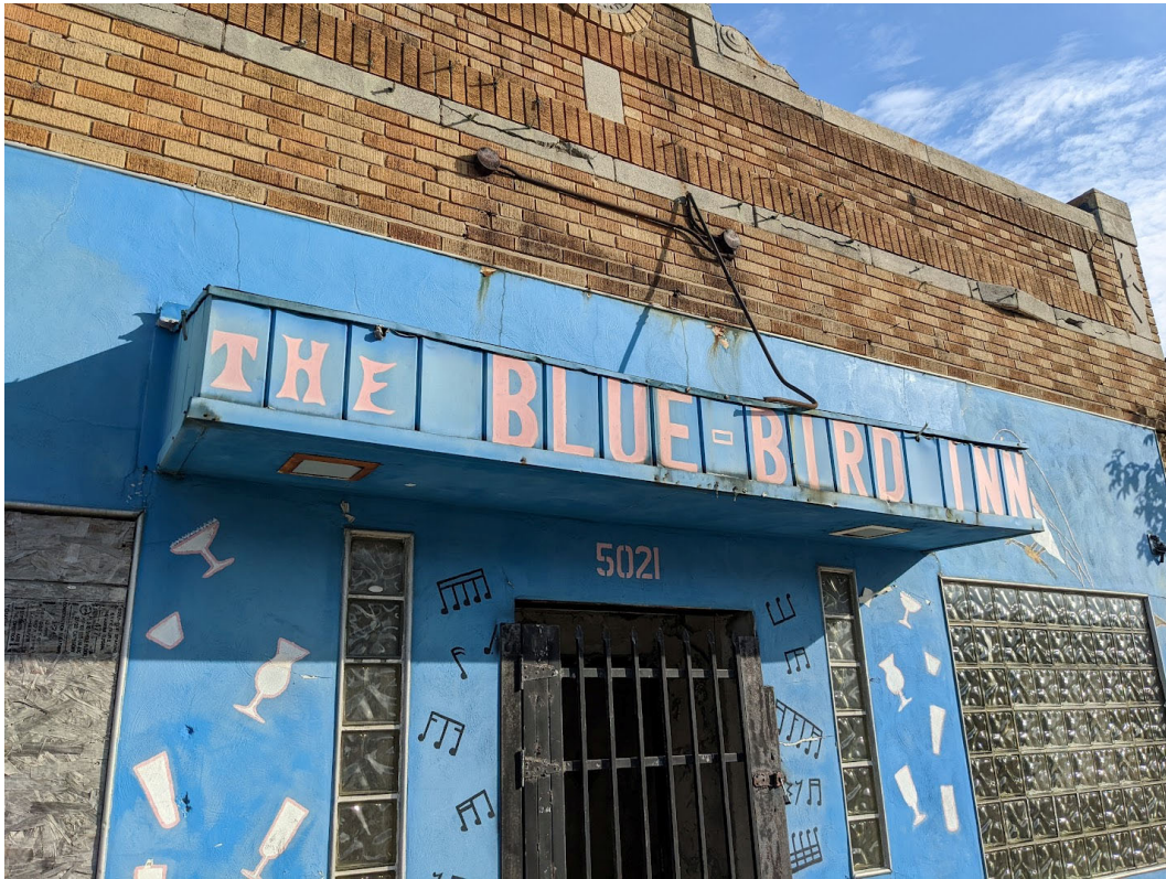
Detail view of 5021 Tireman, at entrance. Staff photo, July 27, 2022.
